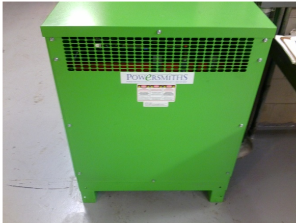
New power efficient transformer GOB
